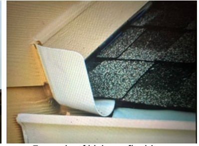
Example of kick out flashing
